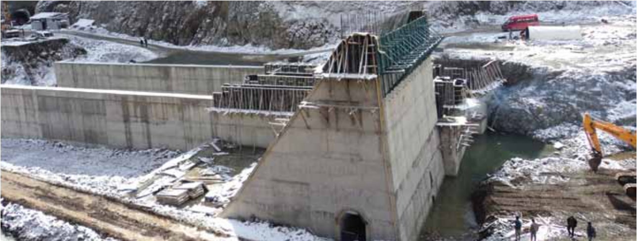
Ayen Enerji Buyukduz HEPP Construction - Elmalı Regulator
